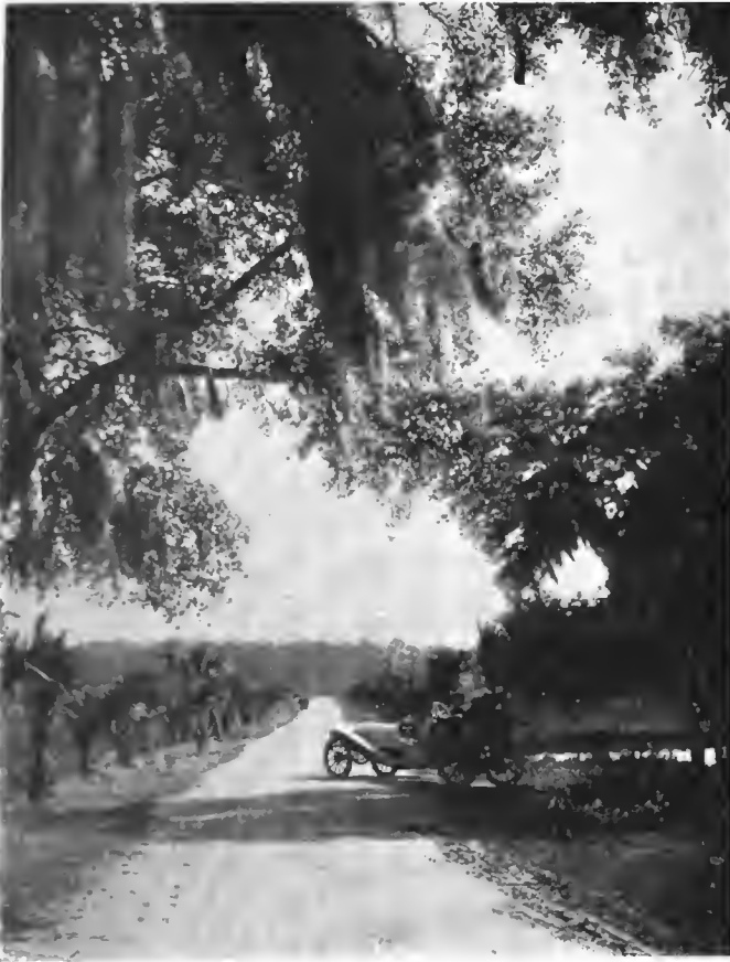
ONE OF THE BEST STRETCHES ON LA ROCHE AVENUE.
